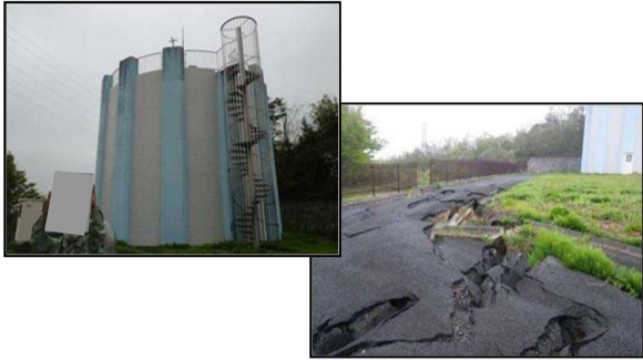
① PC tank installing in area intensity 7 1) L : Complete view of PC tank (with no damage), R : Crack in the surrounding ground
