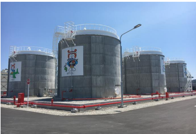
Photo of Completion
