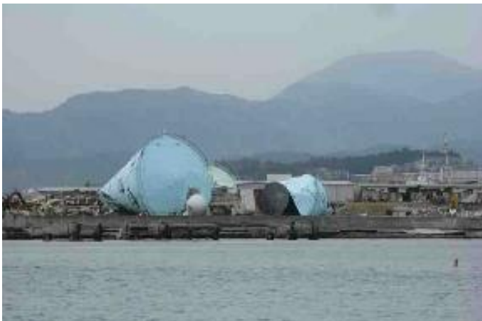
Fuel Facilities Damaged by Tsunami
