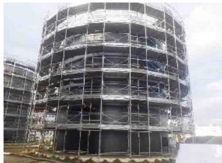
(2) Construction of Steel Tank
