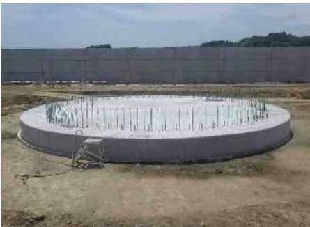
(1) Construction of Bottom Slab
