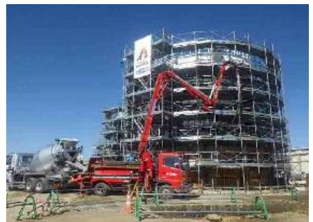
(3) Construction of PC Wall
